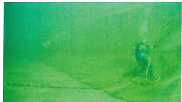
OPG Diver powerwashing to remove algae buildup underwater.
