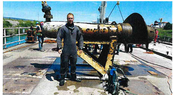
Tempering Water Pump removal
